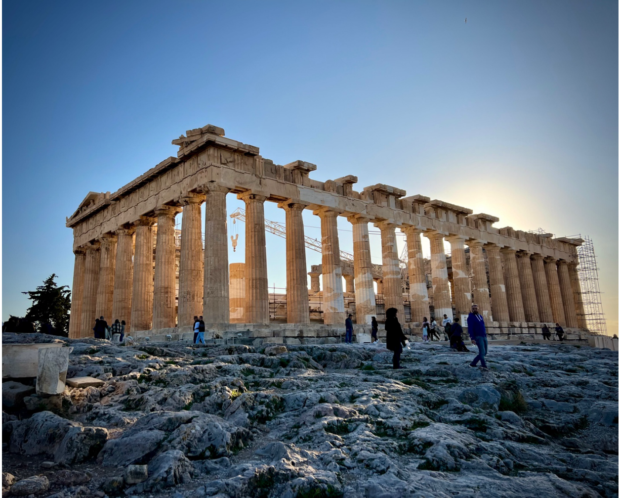
Photo 11. Sun setting on the Parthenon. The lighter coloration within the marble shows areas of restoration, the 17 th -century bombing having knocked down many of the columns. Early reconstruction efforts sometimes cause further damage to the structure. Current efforts are underway to reconstruct the cella (inner chamber) of the Parthenon.
