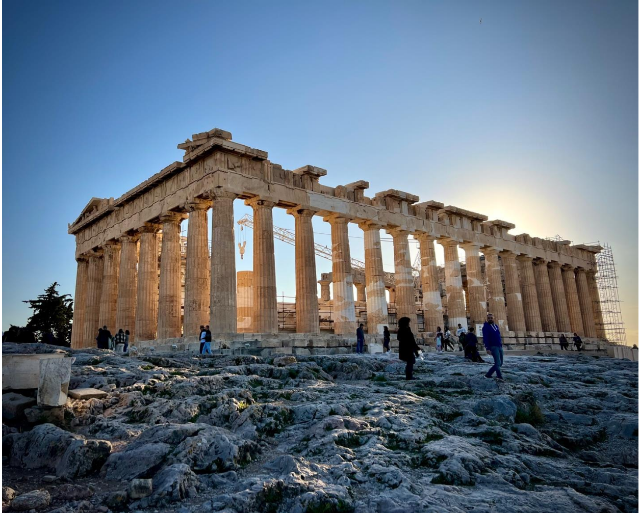
Photo 11. Sun setting on the Parthenon. The lighter coloration within the marble shows areas of restoration, the 17 th -century bombing having knocked down many of the columns. Early reconstruction efforts sometimes caused further damage to the structure. Current efforts are underway to reconstruct the cella (inner chamber) of the Parthenon.
